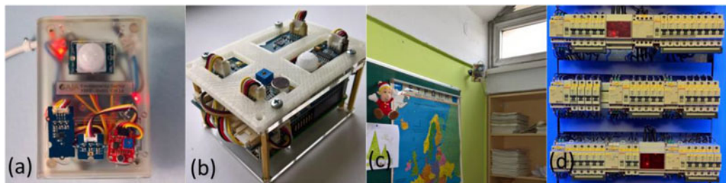
Figure 1. Hardware nodes used and installations inside schools: (a) an Arduino-based node, (b) a Raspberry Pi-based, (c) placement of nodes inside a classroom, and (d) inside an electricity panel.
